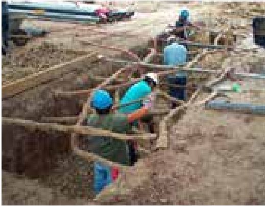
EXCAVATION AROUND EXISTING AND PROTECTIVE WRAPPING OF TREE ROOTS, HERMANN PARK, HOUSTON, TEXAS
